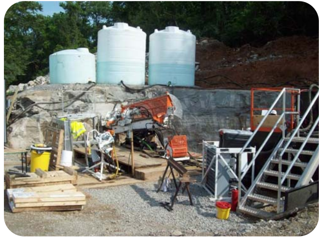
Figure 1 LM 90 Boart Longyear Horizontal Drilling Rig
