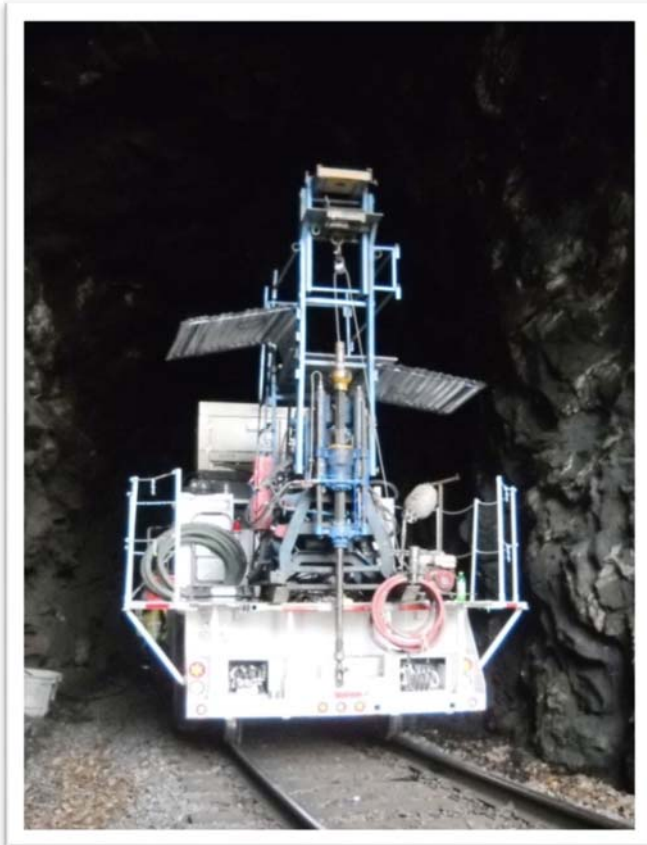
Figure 3 Drilling equipment to be used for vertical and sub-vertical boreholes
